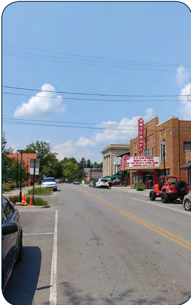
Main Street serves as a minor arterial through Franklin, connecting the downtown to areas north of the city along US 31
