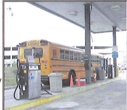
This fueling island is roofed and absorbent materials are provided in case of spills. However, the used absorbent hasn't been swept up and disposed of properly
