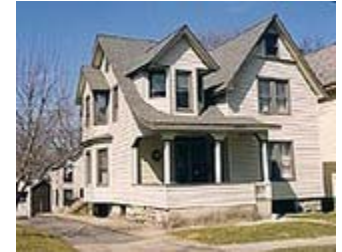
When vinyl was installed on this Victorian home, the architectural details were covered.
